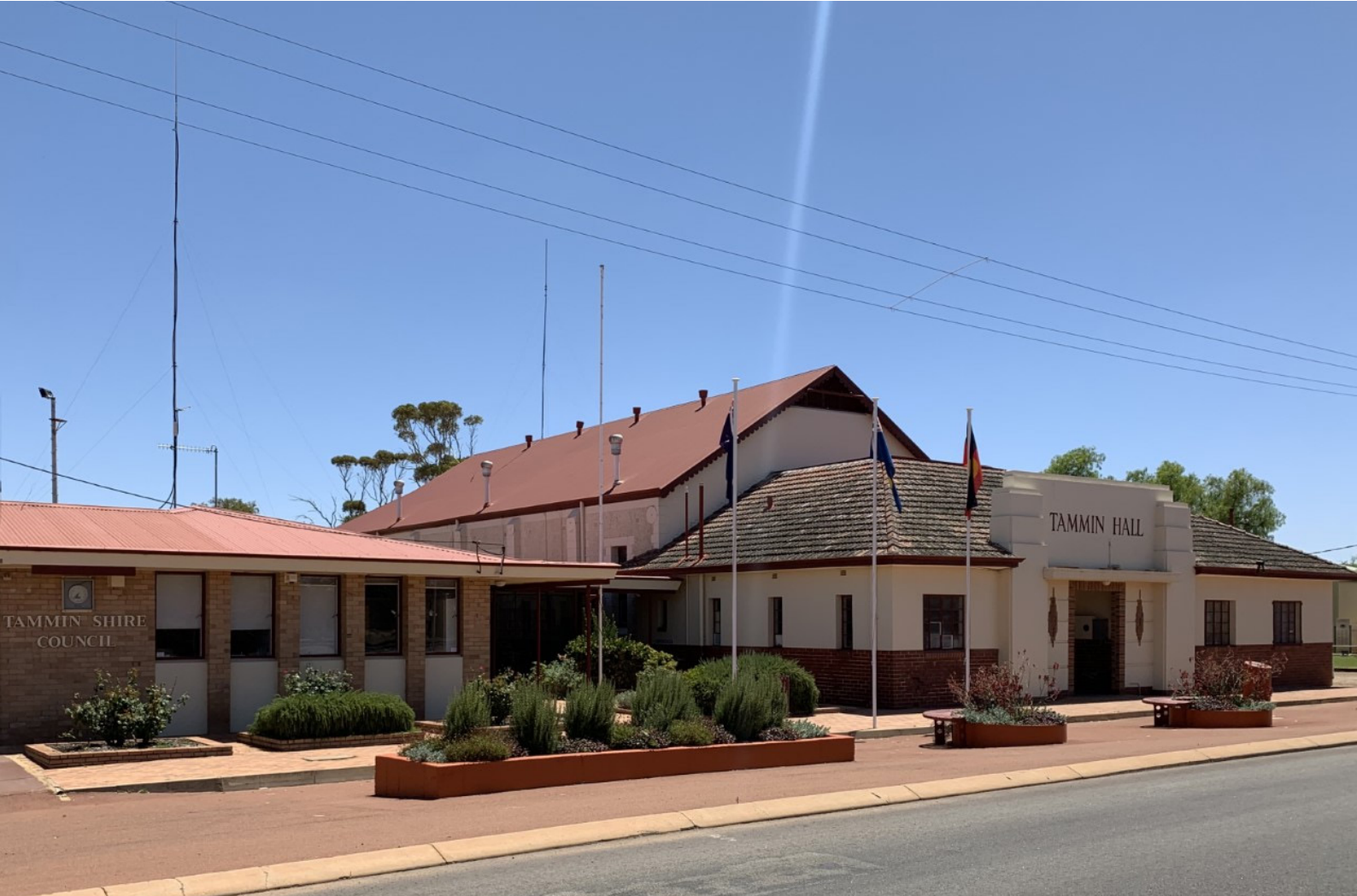
Above: The Tammin Town Hall built circa 1911. The Hall is a significant focal point and public venue for residents of the Shire of Tammin.
