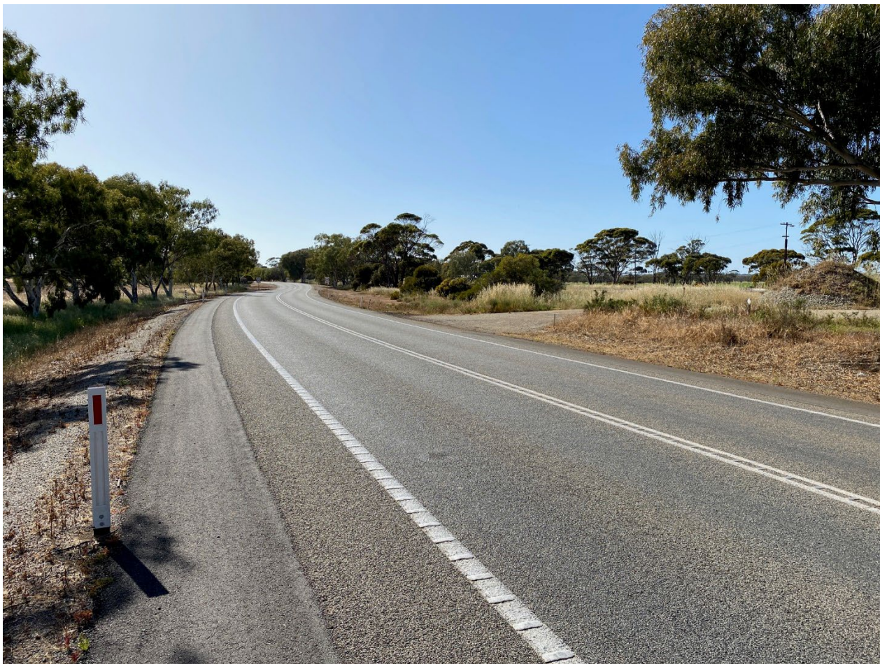
Photograph 3 - View South-East across Great Eastern Highway to Existing Eastern-Most Crossover
