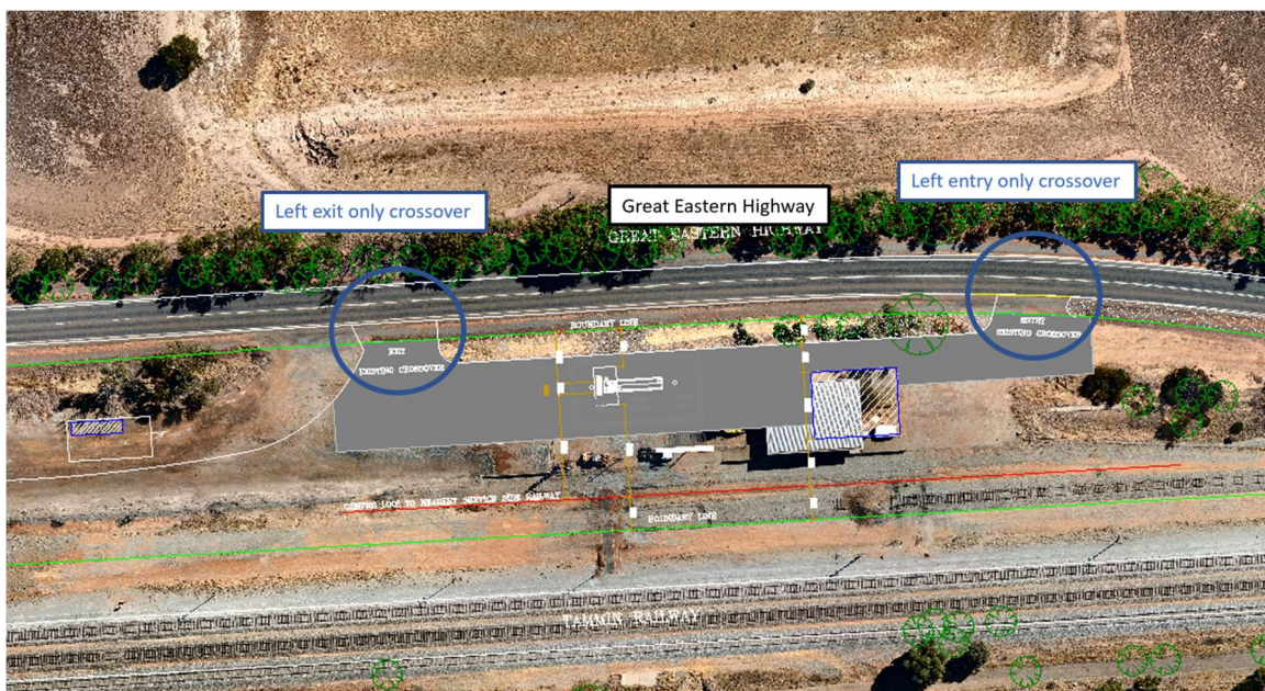
Figure 3: Subject site with crossover location
